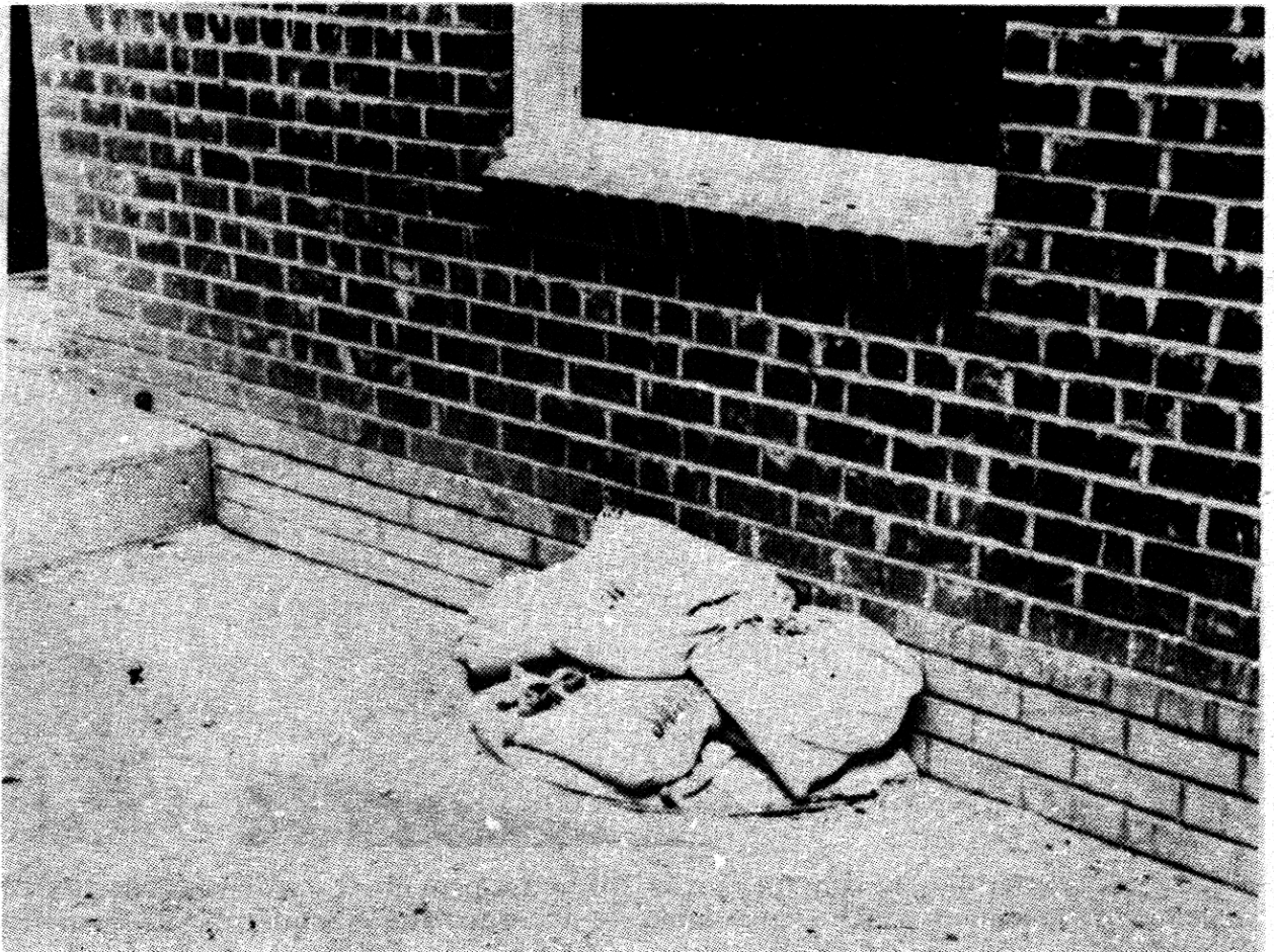
Cellar window, two-story brick house, sandbagged
